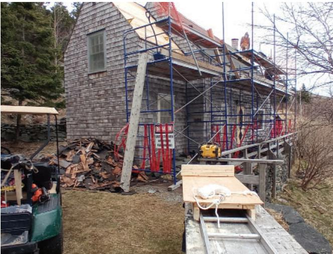
It is now nearing the end of April and Kent Cottage is getting ready for its new roof, roof number seven. With the help of Aaron and Byron Rodway of Rodway's Excavating and contractor, Anthony Nofle, the south side of the cottage is enmeshed in scaffolding. Jake's old cedar shake roof has been taken off and piled on the ground and a protective layer of Ice and Water Shield applied to the roof boards. Until we complete the wood shingling, this underlayment will keep out the water.
