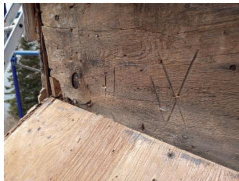
The old lead flashing between the shed roof and the wall was deteriorated and in order to replace it I had to remove three courses of wall shingles and expose the old sheathing boards, probably from the 1830s. The exposed board was sawn with a pit saw and these marks may have identified the sawyers so they could be paid for their work.
